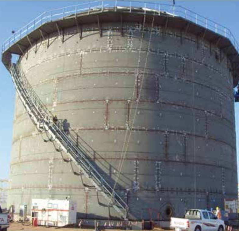
Chemical Storage Tank
